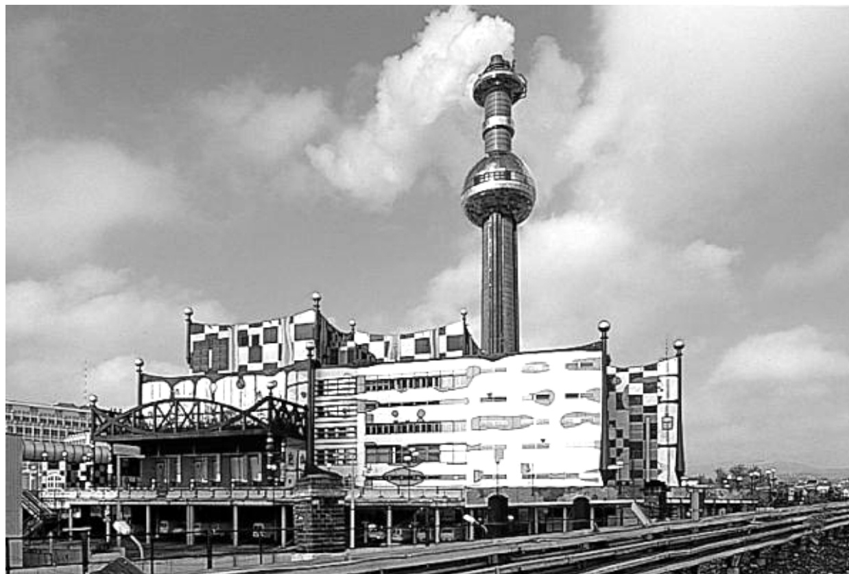
Figure 8 WTE plant Spittelau Vienna
